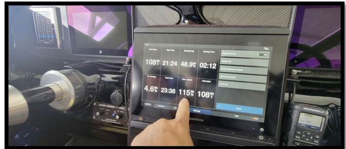
Reviewing the teams' electrical equipment.
